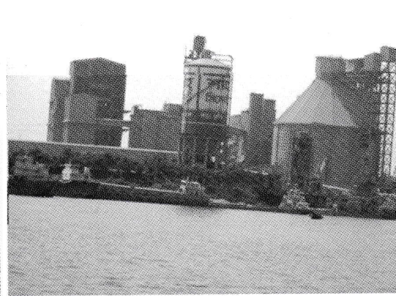
Photo 3.3: Cement Factory Pollutes Dhaleshwari River
