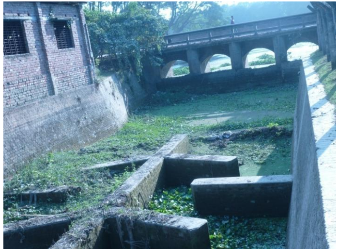
Photograph 3.1: The water regulator structure - fish by pass and sediment trap (British design) at the mouth of Kata Khal joining the Kobadak at Jhikargacha.
