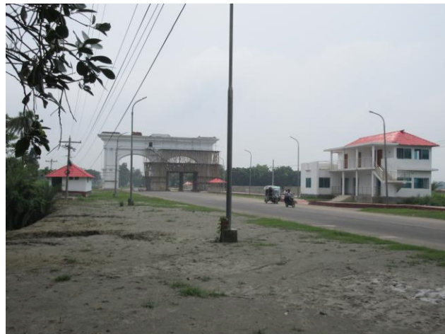
Photograph 10.4: Benapole Gate under construction
