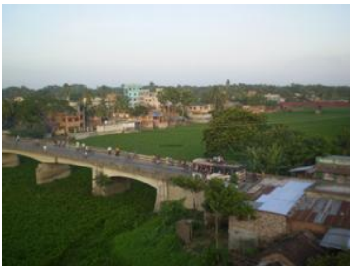
Photograph 10.1: Jhikorgachha Bridge over Kobadak
