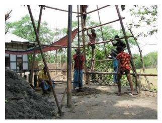
Figure-1: Drilling Procedure of Monitoring well.
