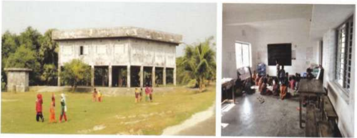
Figure 3 Cyclone shelter in Char Gangamati is used as educational institution in normal time. (Mowla&Kabir, 2012)
